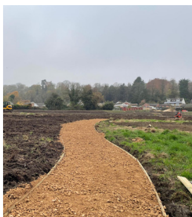
Surfacing in progress
